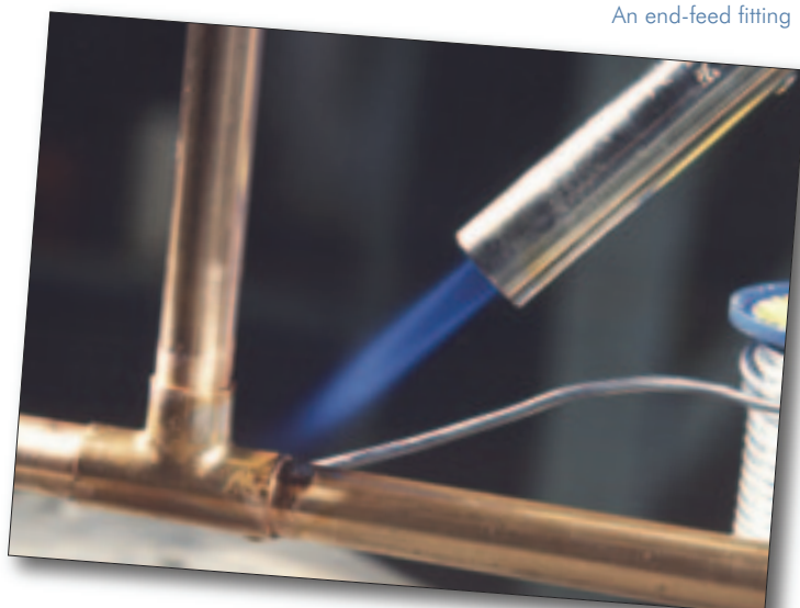
An end-feed fitting
